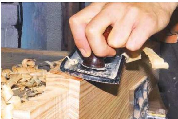
The parts of the door most vulnerable to rain are the tops of the rails where water might sit and seep into the joints. To preempt this they sloped them. With no machine interested in doing this, they reverted to a jack plane
